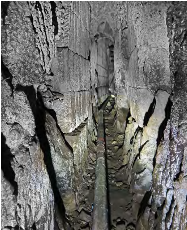
Beyond the debris barrier of the Nemi drain. The underground junction between the Roman entrance chambers and the mountainside
